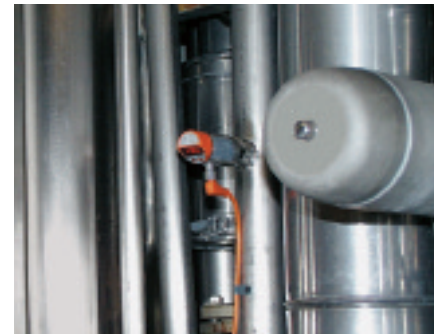
A rotatable display allows the process temperature to be viewed from any angle.
