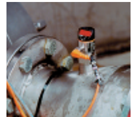
The PN pressure sensor monitors line pressure in a pipe and provides 4-digit numeric indication.
