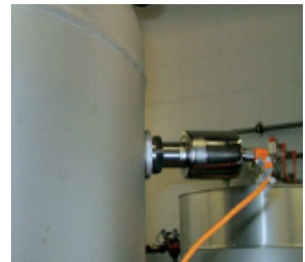
The TAD transmitter provides a switching output to indicate when a drift occurs. The warning and alarm levels are configurable.
